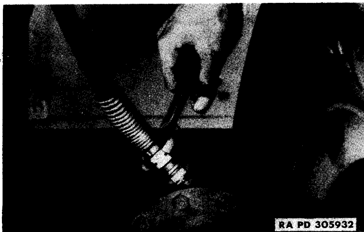
Figure 115—Installing Brake Line at Diaphragm
