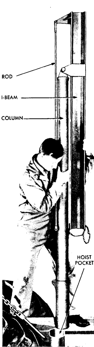
INSTALLING HOIST COLUMN IN HOIST POCKET—STEP 2
