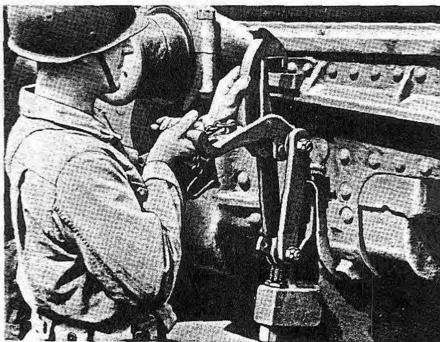
Figure 84 – Detaching Locking Hook From Cradle
