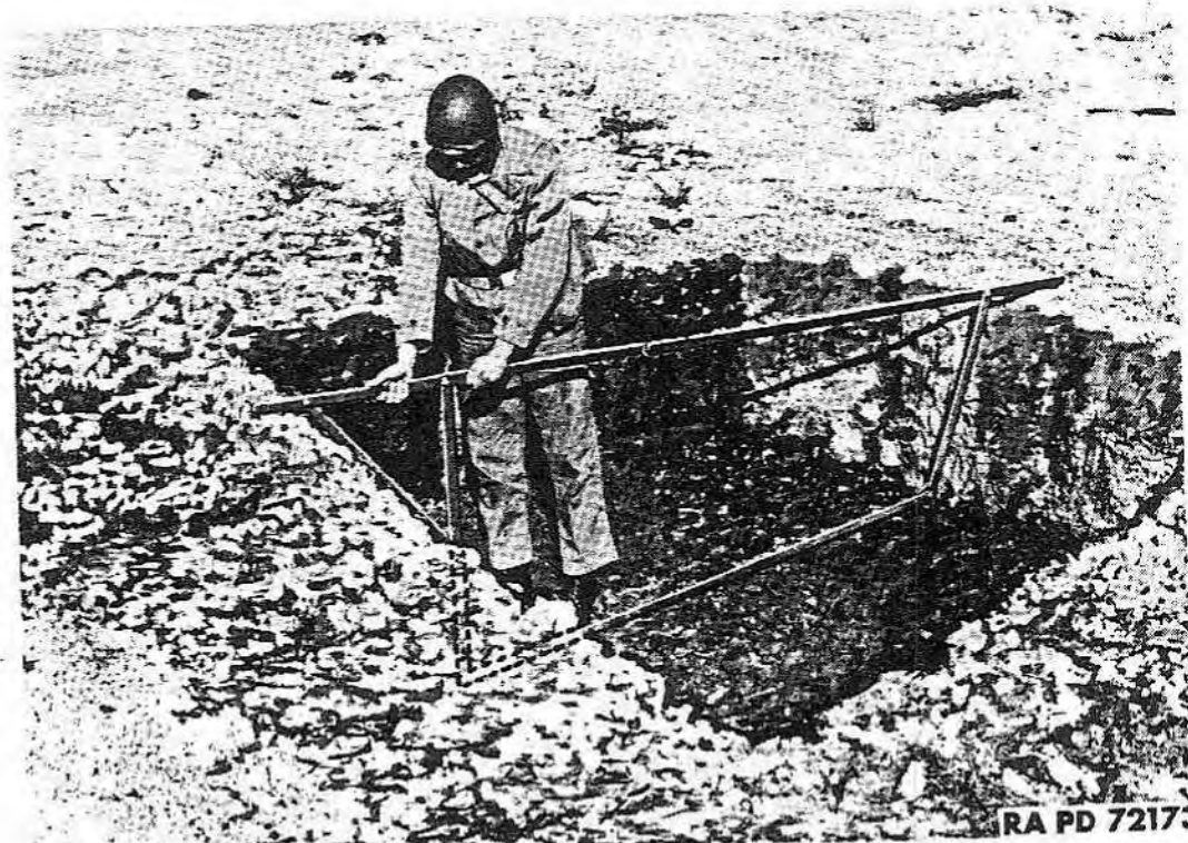
Figure 73 — Checking Shape and Depth of Pit With Templates Nos. 2 and 3
