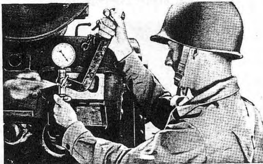
Figure 123 – Checking Liquid Level in Recuperator Reservoir
