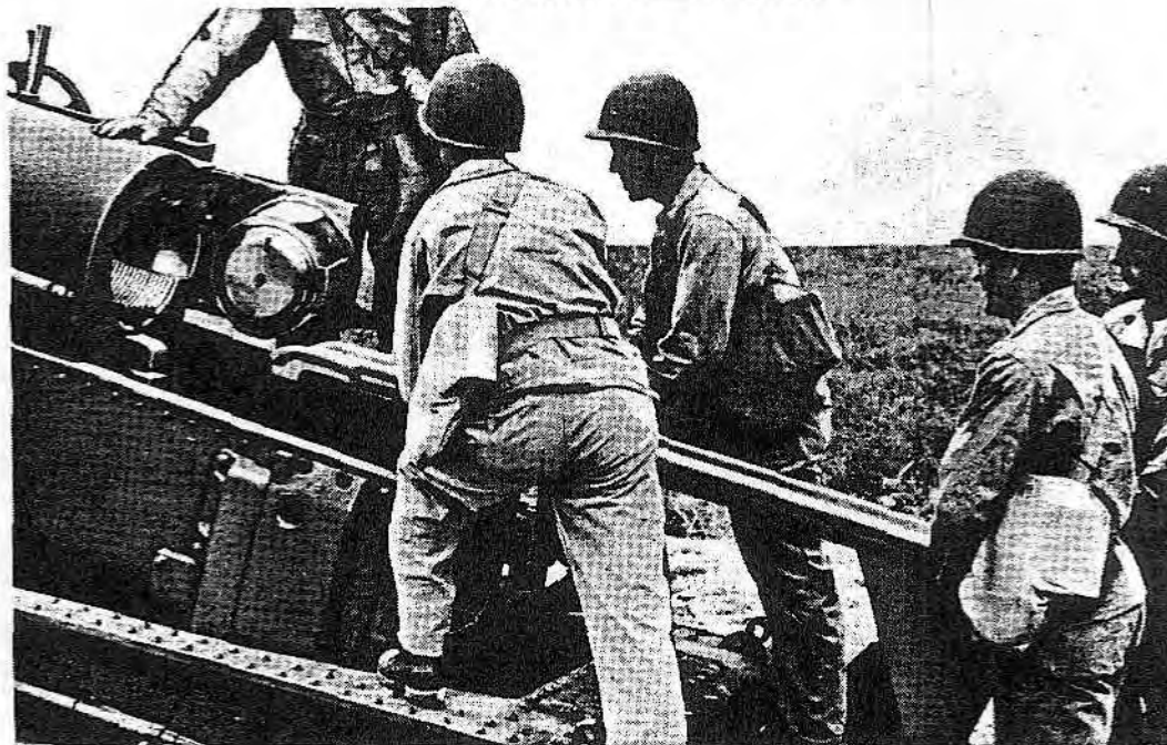
Figure 96 – Installing Loading Ramp
