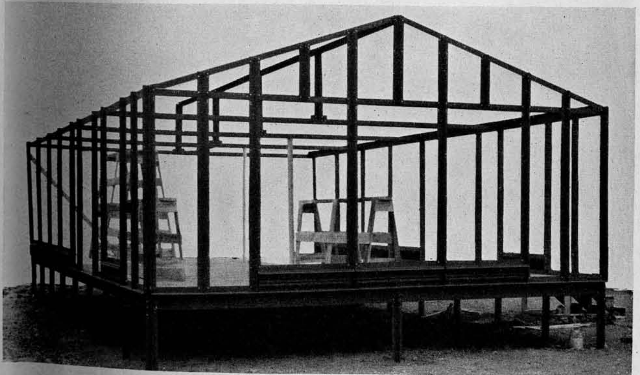
Figure 27. Wall framing completed.
