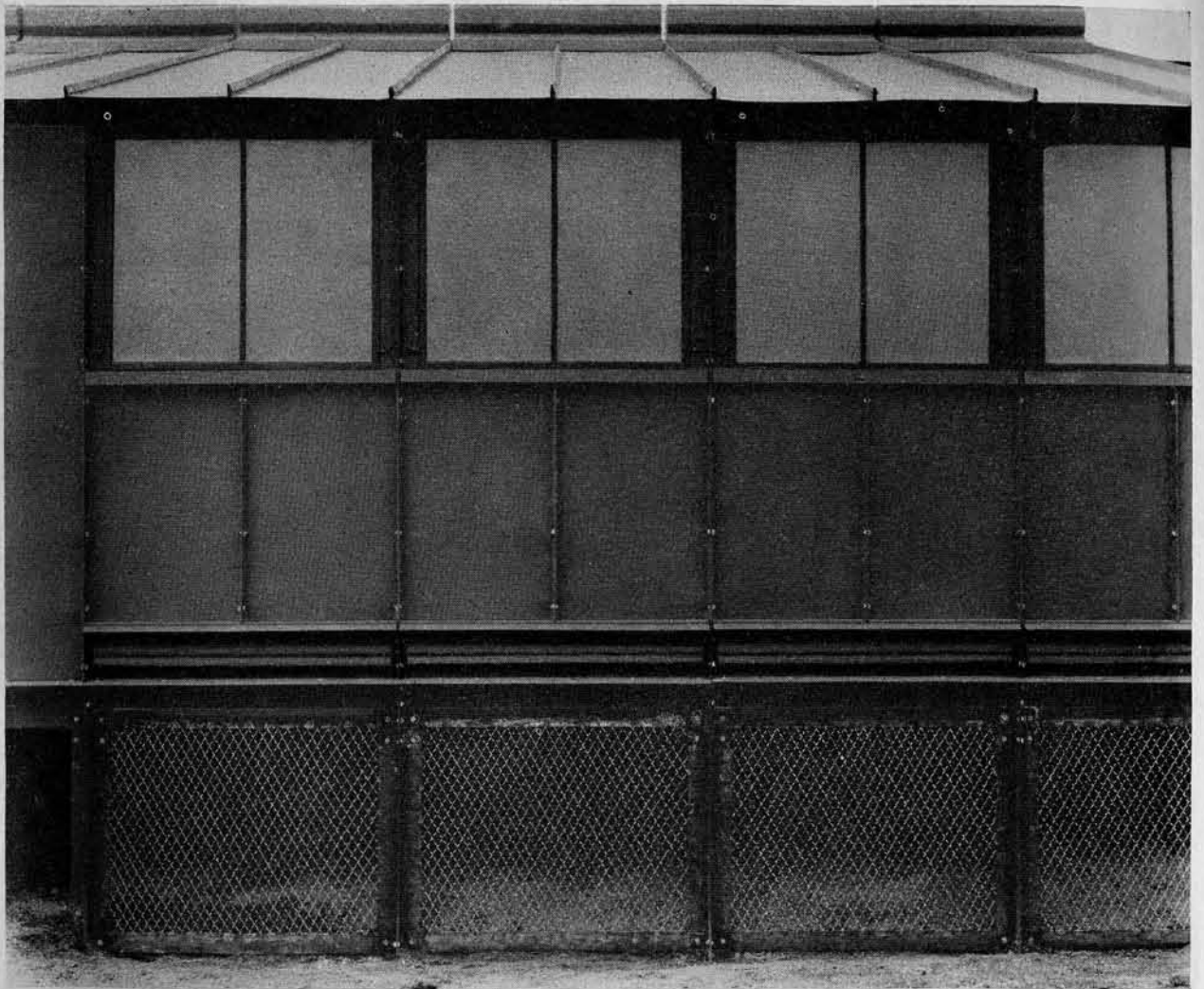
Figure 31. View of completed exterior side wall.
