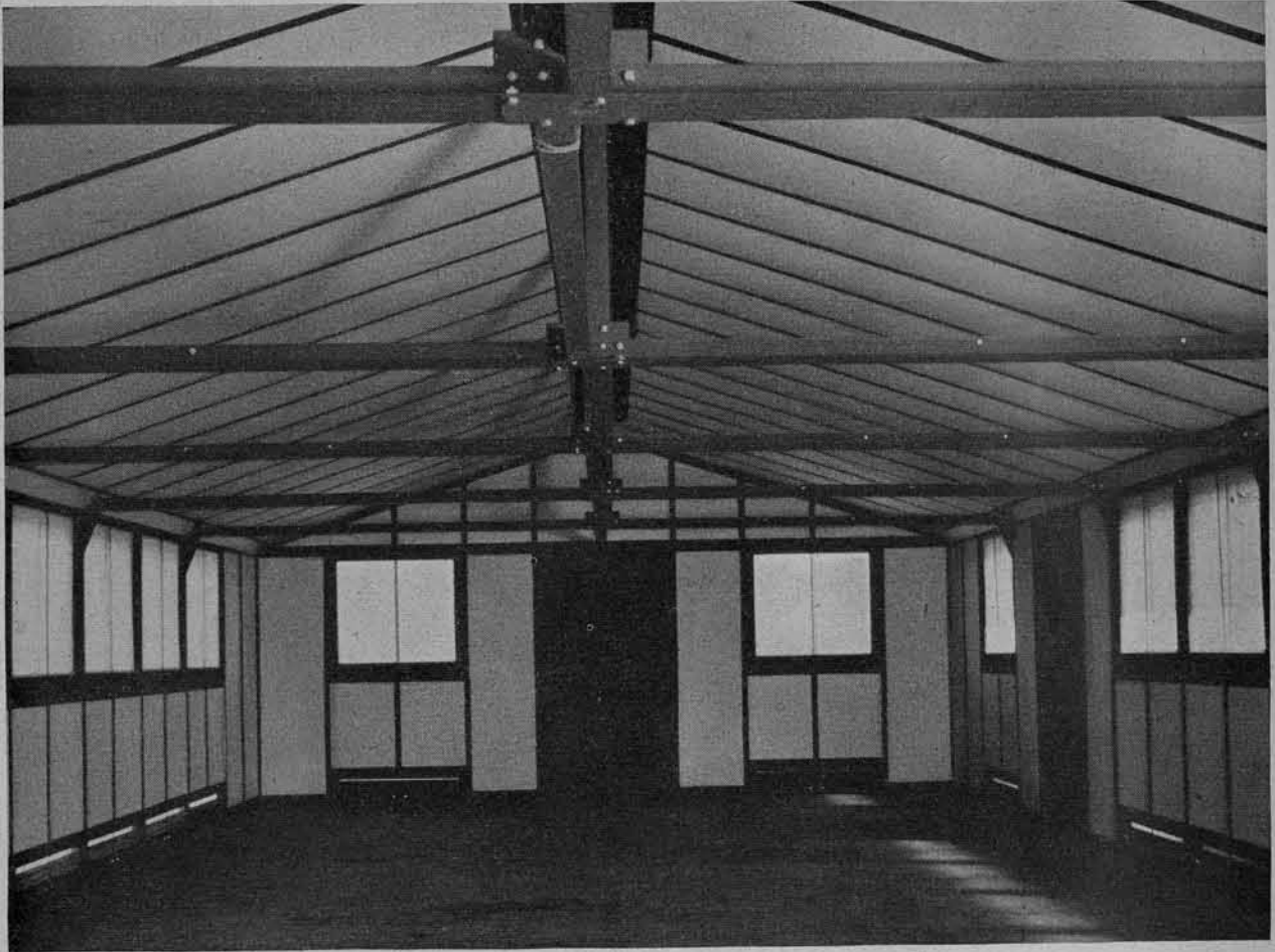
Completed interior of office building before installing partitions.
