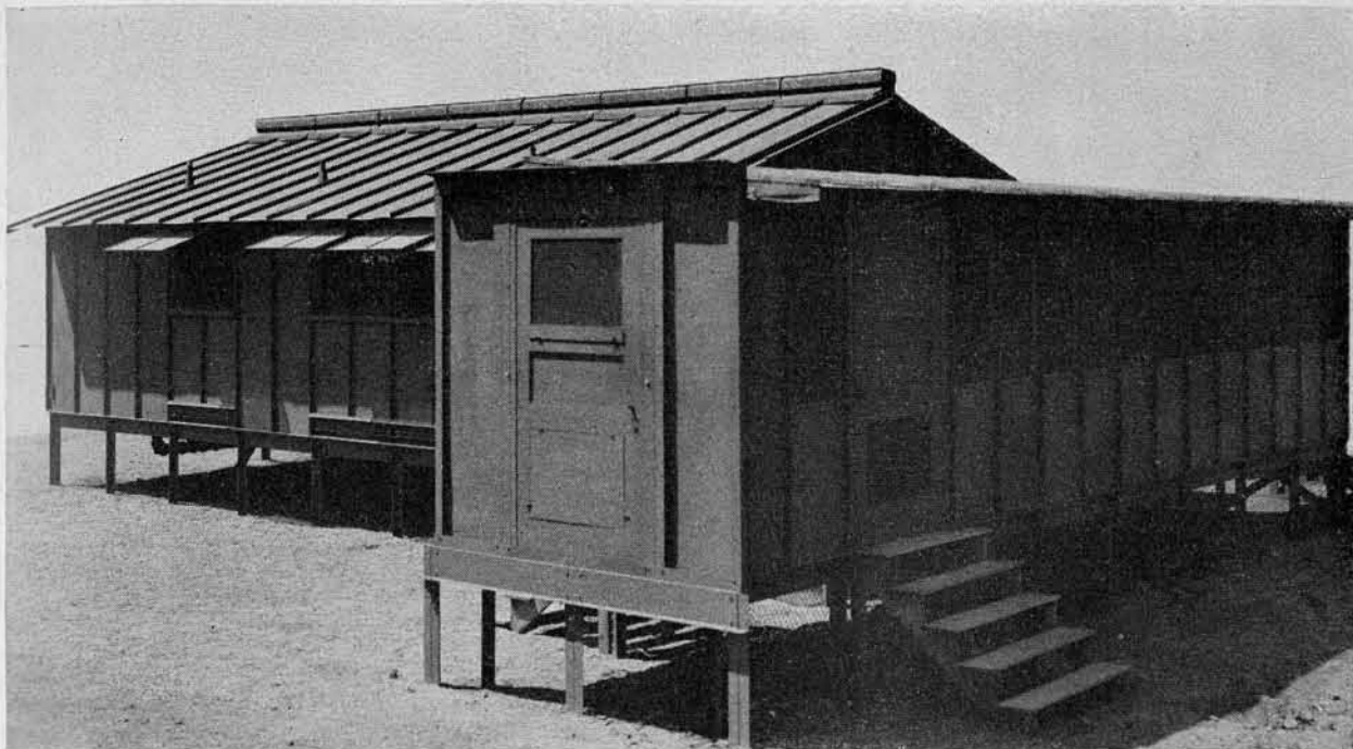
Figure 52. View of completed corridor from exercise yard.
