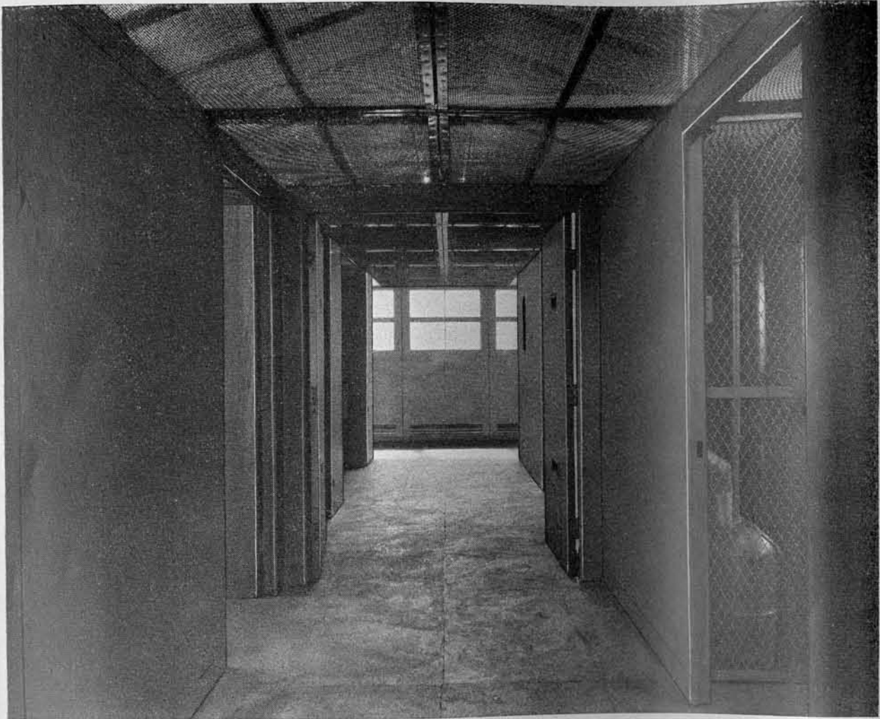
Figure 51. Interior view of completed utility building.
