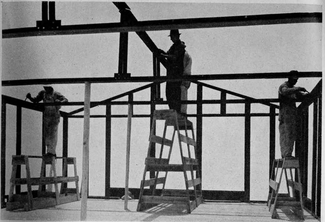
Figure 26. Erecting trusses and showing suggested platforms.
