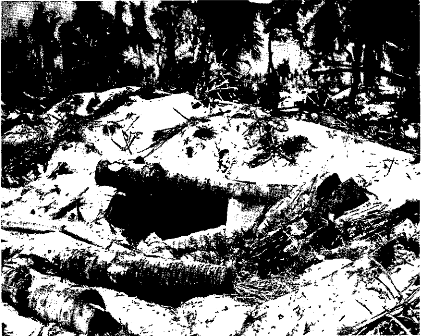
Figure 34.—Gunport in Japanese log and sand pillbox on Betio.
