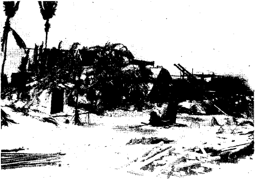
Figure 42.—8-inch gun emplacement on southwest point of Betio island. Note camouflage and sand-banked concrete revetment.
