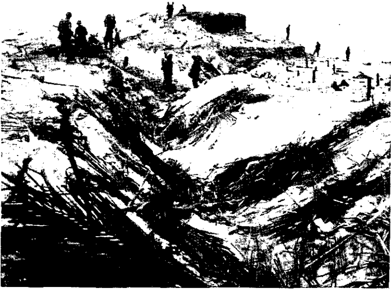
Figure 28 (a).—Rear view of heavy concrete circular pillbox on Roi. Note camouflaged communications trench.
