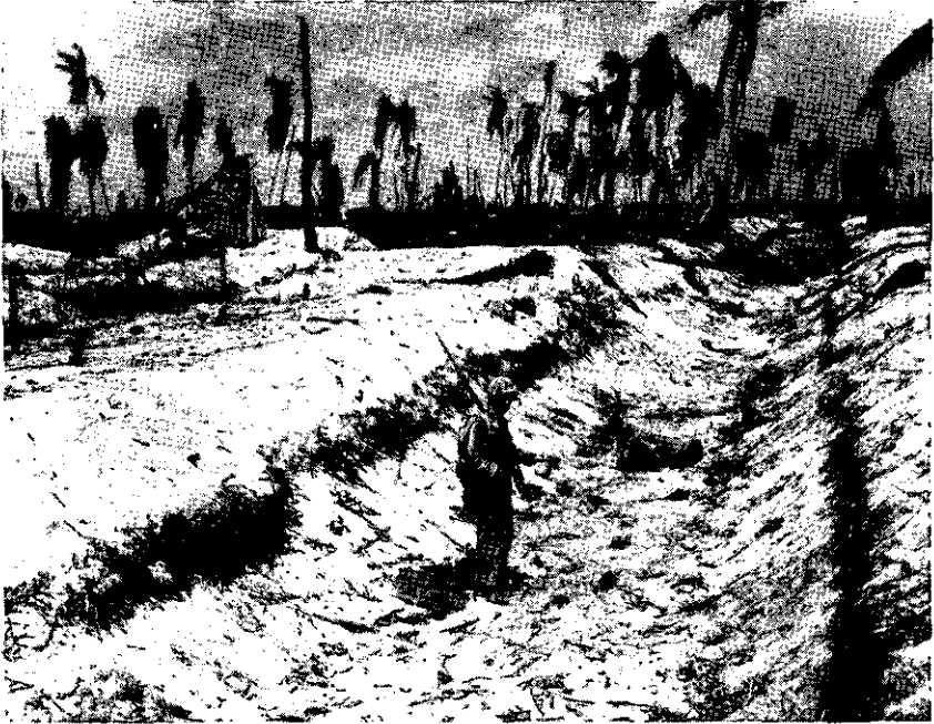
Figure 26.—Tank trap just off a Betio beach.
