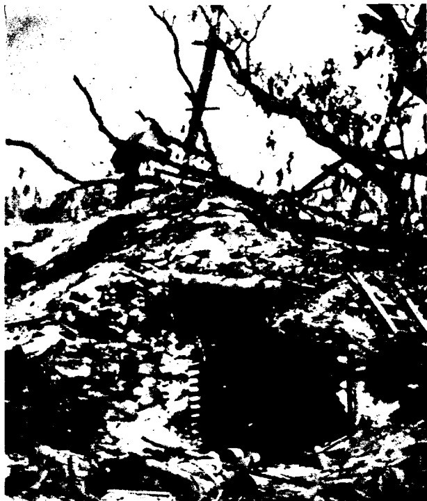
Figure 112. Entrance to pillbox on Tarawa.
