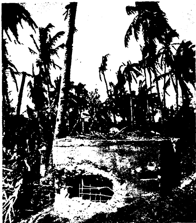
Figure 109. Concrete pillbox on Guam.
