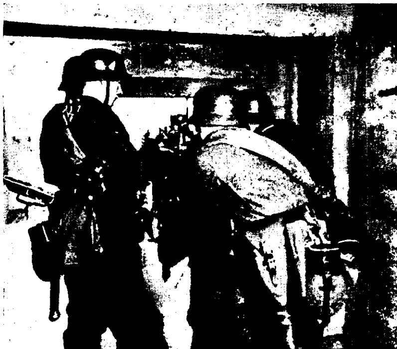
Figure 20.—Machine-gun embrasure (interior view).
