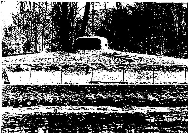
Figure 26.—Work with cupola, embanked.
