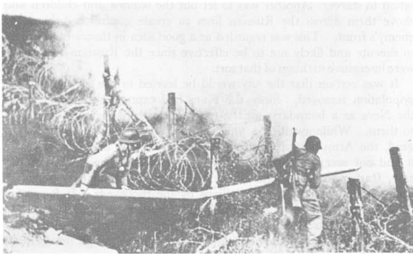
Finnish engineers using bangalore torpedo to demolish Russian fortifications on the Isthmus of Karelia.
