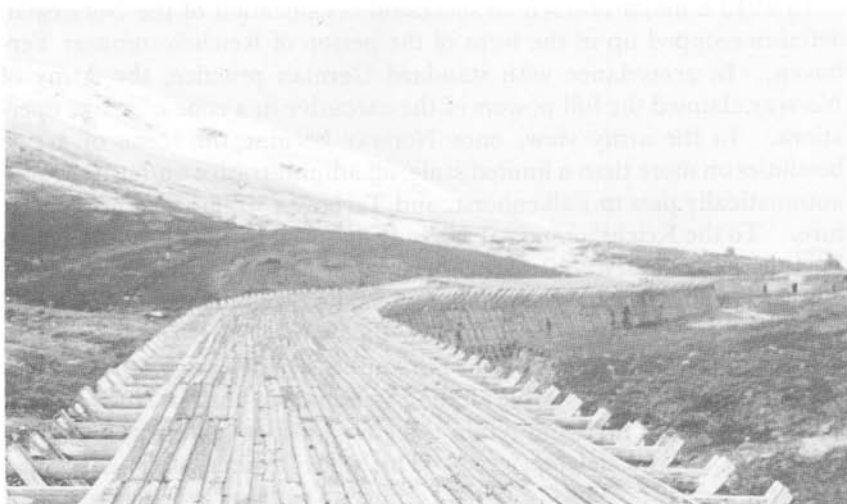
Snow tunnel on Reichsstrasse 50.
