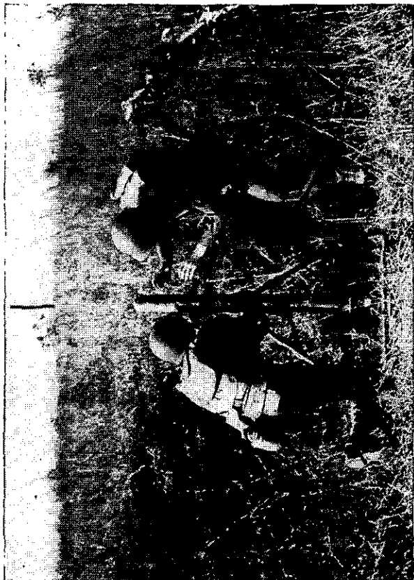
NOTE.—Heavy grass provides some concealment from aerial observation. FIGURE 48.—81-mm mortar set up on reverse slope. Aiming stake is on crest.
