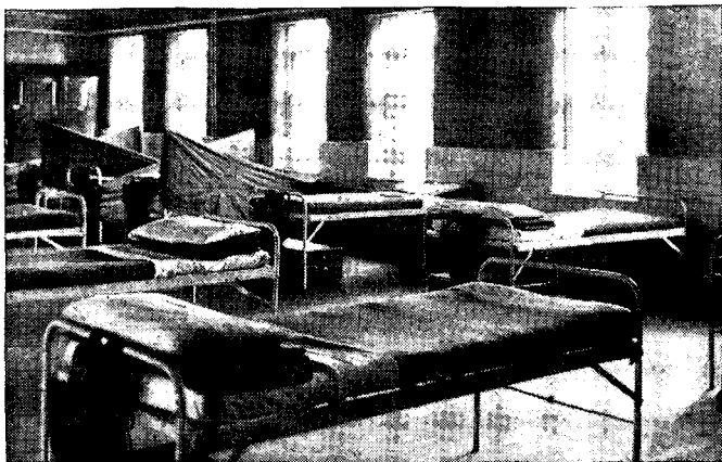
FIGURE 5.—Method of constructing cubicles in squad rooms by the use of shelter tent halves with head and foot arrangement of beds.
