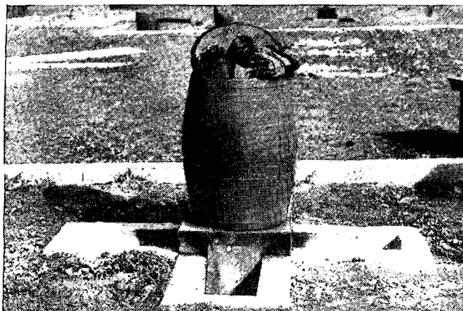
FIGURE 66.—Disinfestor, Serbian barrel type.
