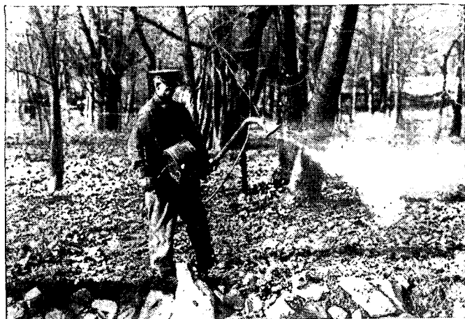
FIGURE 60. Method of producing dust cloud of paris green larvicide with hand-operated dust blower.
