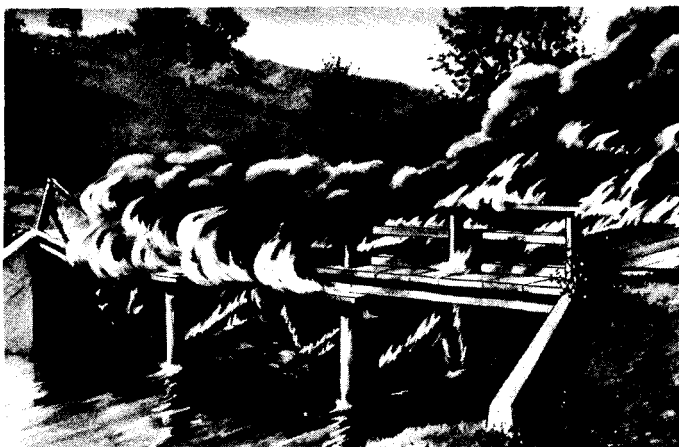
Figure 37. Economize on explosives by using expedients. This method is time consuming and often ineffective. Destruction must be carefully checked.
