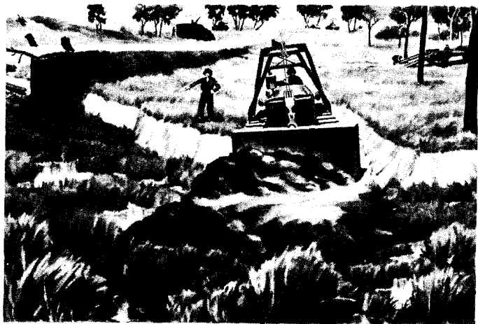
Figure 22. Save time by having power equipment available.
