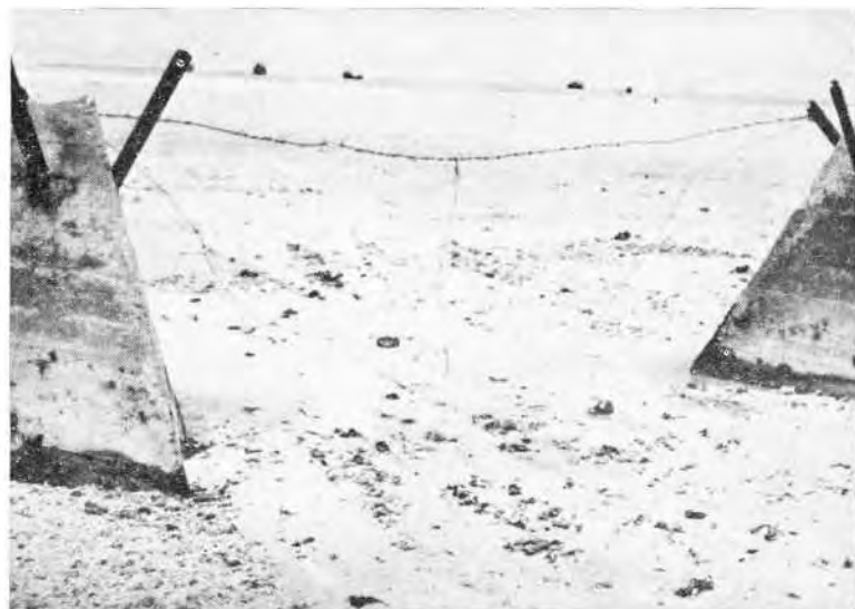
Figure 24. Here is a typical trap which you are likely to encounter on the beach. Notice the three trip wires hooked to the barbed wire. The explosive charge is buried under the sand. (This is a photograph of an actual trap found at Tarawa.)
